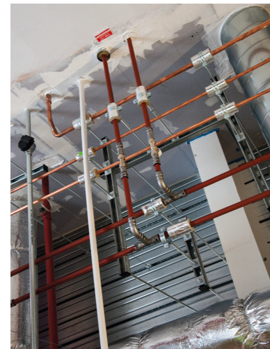
Viega's SC-Contur technology provides a 100% positive leak should a connection be inadvertently unpressed.
