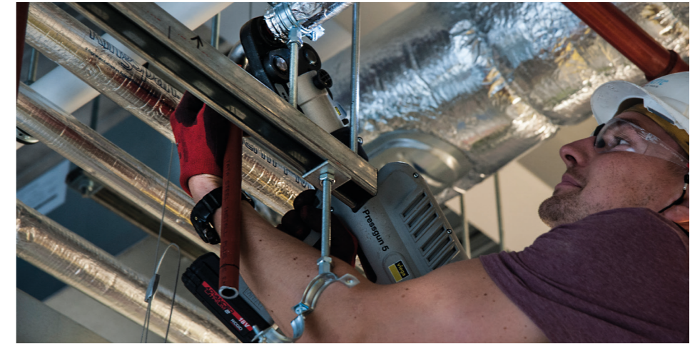
Megapress connectors are pressed easily, quickly and safely using Viega's Pressgun 5 machine.
