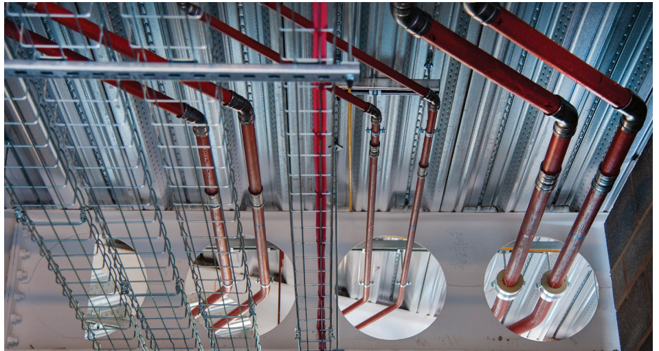
Viega's SC-Contur technology provides a 100% positive leak should a connection be inadvertently unpressed. This can be easily spotted and rectified during testing.
