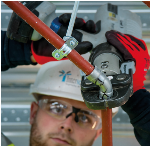
Megapress connectors are pressed easily, quickly and safely using Viega's Pressgun 5 machine.
