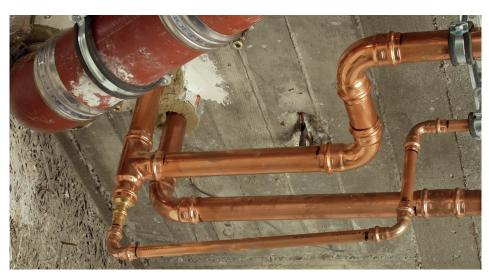
Copper was the material of choice for the heating and water pipework, selected from Viega's Profipress range.
