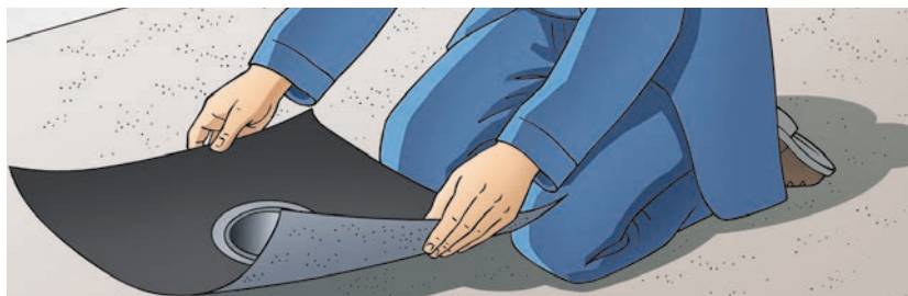
Fig. 3 – 19 Arranging the sealing collar
