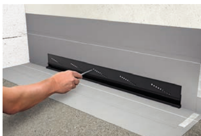
Fig. 3 - 31 Wall drain - sealing flange
