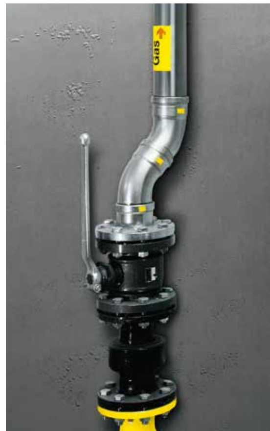
Sanpress Inox G XL – flexibility for gas installations in industrial applications.
