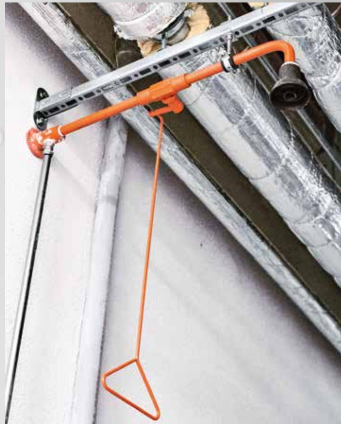
Body shower made with Sanpress Inox in meat product manufacturer Metten's production facilities.
