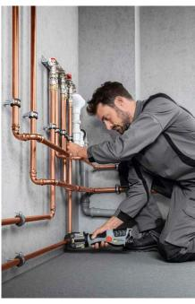
With its inline design, the Pressgun Picco 6 Plus also allows users to work parallel to the floor
