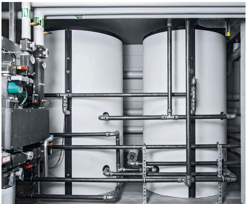
Megapress in a heating installation with energy buffering.
