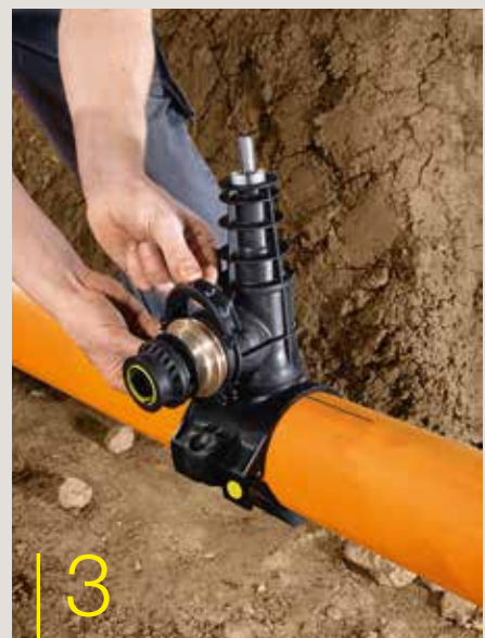
3 Insert and secure the connecting piece.
