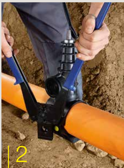
2 Press the fitting with the manual tool or Pressgun.
