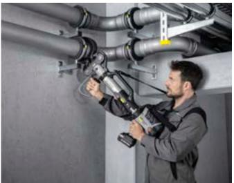
With dimensions of up to 2 inches, the Megapress S press connector system provides the best possible connection option to local and district heat supply systems (in accordance with AGFW FW 524). From the point of entry into the building, the thick-walled steel pipes that are frequently used in these areas can be pressed together quickly and safely.
