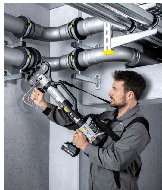
With the Pressgun 6 Plus – shown here in combination with the Press Booster for Megapress XL dimensions – Viega press connector systems can be pressed easily, quickly and safely.
