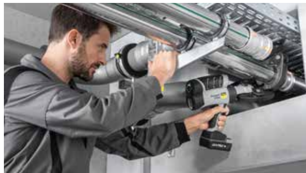
The Pressgun 6 Plus makes it possible to carry out single-handed pressing of XL dimensions.
