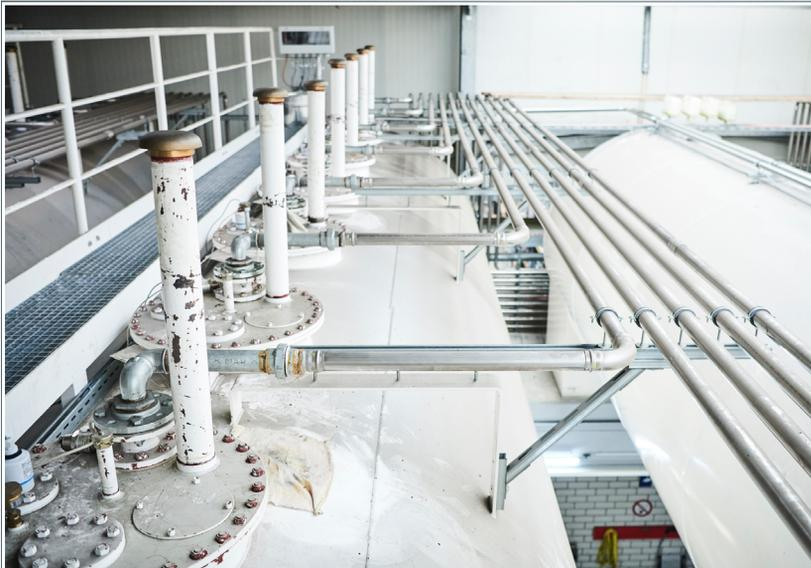
Fig. 174: Cooling lubricant tanks filled and emptied using Viega Sanpress Inox G
