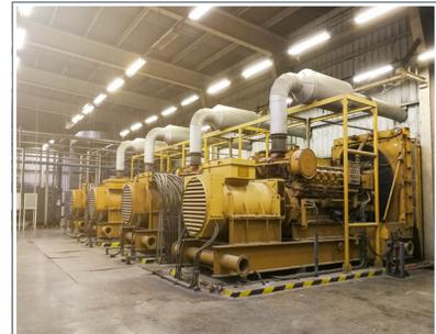
Fig. 170: Diesel-operated emergency generator
