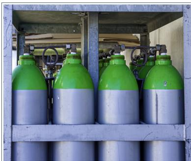
Fig. 147: Secured liquid gas cylinders
