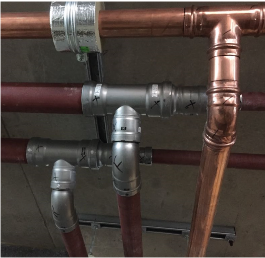
Copper was the material of choice for the hot and cold water pipework, selected from Viega's Profipress range.
