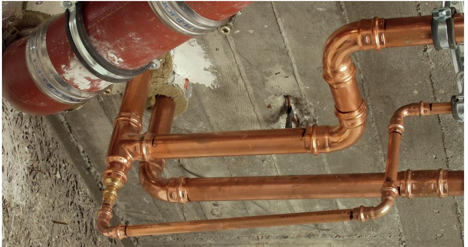
**Copper was the material of choice for the heating and water pipework, selected from Viega's Profipress range.**
