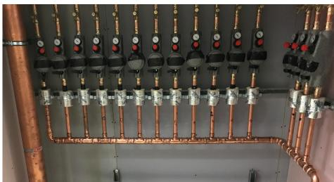
Viega's copper Profipress system was used extensively with a size range from 12 to 108mm.
