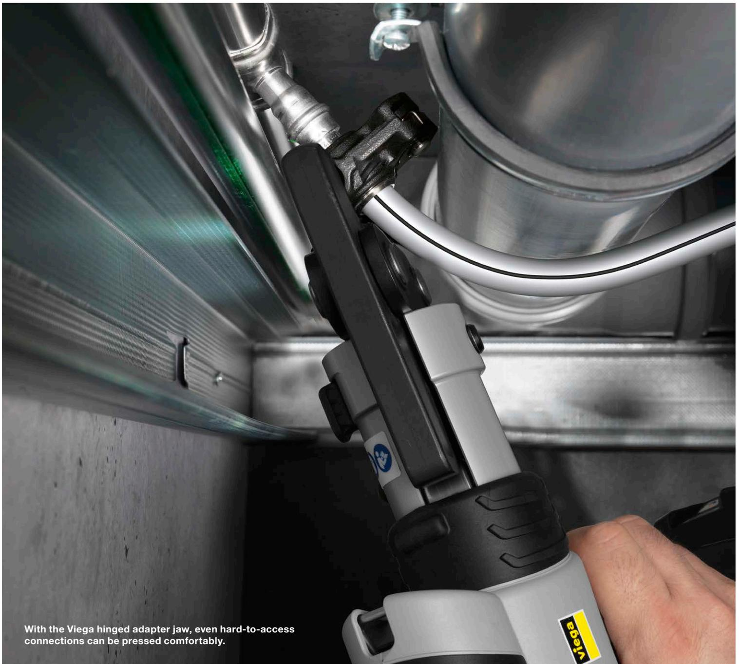
With the Viega hinged adapter jaw, even hard-to-access connections can be pressed comfortably.
